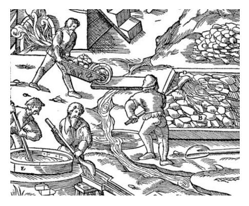
**Figure 1.** "The rocks are . . piled in . . heaps fifty feet long, eight feet wide and four feet high, which are sprinkled for forty days with water. The rocks begin to fall to pieces like slaked lime, and there originates a . . new material". Drawing and text from De Re Metallica, Herbert Hoover translation, published by Dover Publications, Inc.
