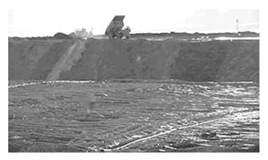
**Figure 5** Truck dumping an upper 10 meter lift of run-of-mine ore on top of a lower lift that has already been leached.
