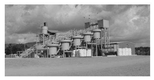
**Figure 9** Five-stage carbon adsorption column plant (CIC plant) at Glamis Gold's San Martin, Honduras project. There are two parallel column trains (one is behind the other in this view). The plant can process up to 900 cu m of solution per hour, and is sized for an operation that processes up to 20,000 tonnes of ore per day.
