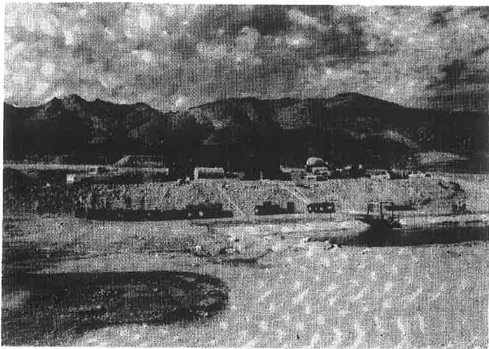
Figure 11. Individual pregnant ponds are below the heaps. From there, solution is pumped through the recovery trailer, and is then discharged to the barren pond in the right foreground. Solid caustic soda and cyanide are manually added to the barren pond before solution is recycled to the heaps.
