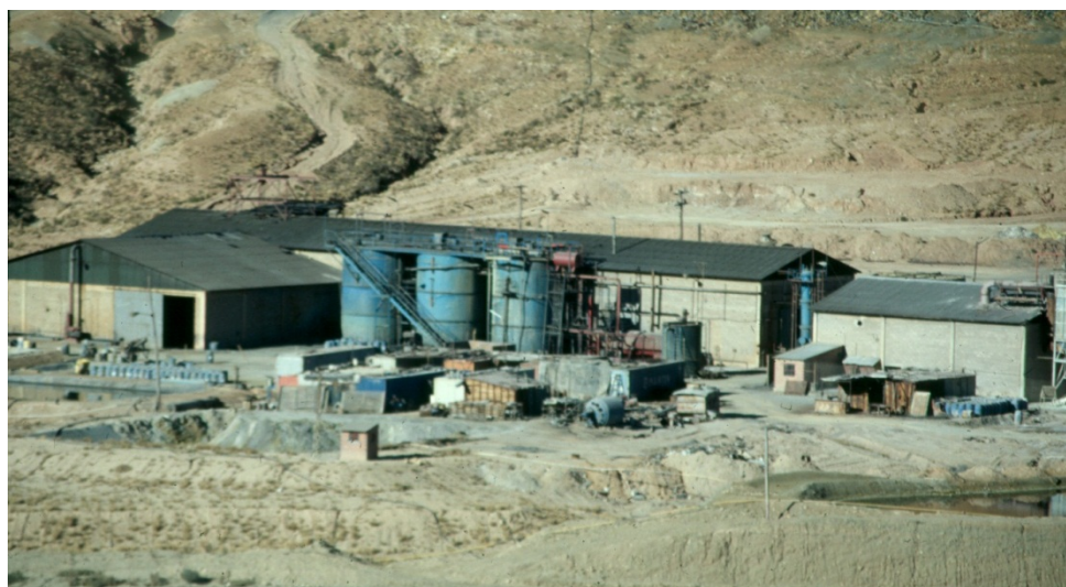
Figure 1. The 600 tonne/day Itos Bolivia chloride leach plant for silver. Leach tanks can be seen in the center of the photo. The tailings filter building is on the left, process building in the rear, and the pyrometallurgical plant on the right.
