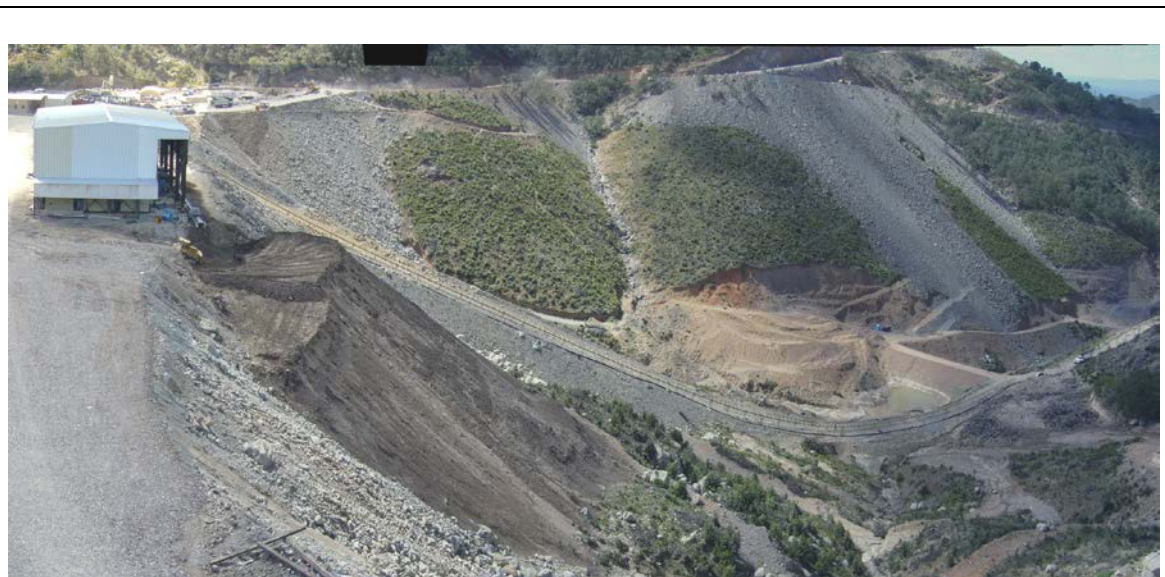
FIGURE 3. TAILINGS FILTER BUILDING AND TAILINGS CONVEYOR
