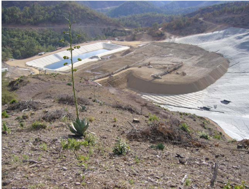
FIGURE 5. IN THIS EARLY PHOTO, THE PATTERN OF SPIRAL STACKING IS JUST BEING ESTABLISHED
